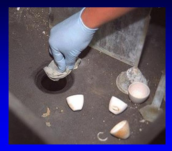
All visible mercury beads are collected using the mercury vacuum followed by specialty wipes.
